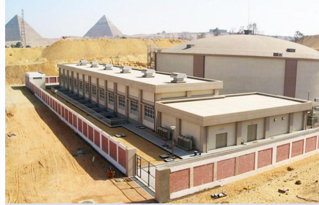
Water Supply & Sewerage Project, Giza, Egypt
